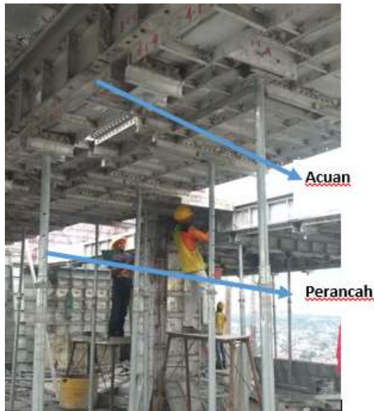
Gambar 1. 1 Bekisting Aluminium
